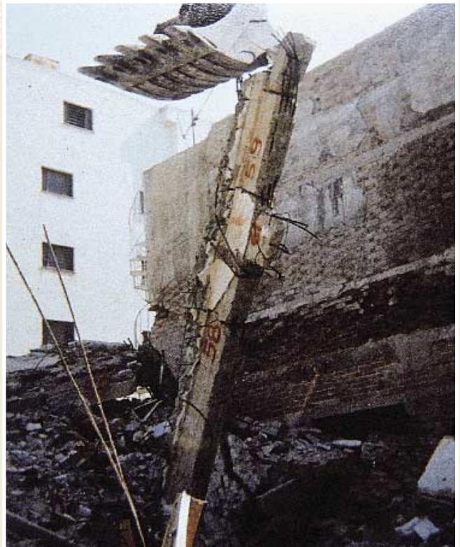
Photo 9-10: Elevation of a slab (photo 9) and a beam element (photo 10) by a shovel excavator. Eccentric fastening so that the main reinforcement takes a vertical direction and therefore the folding of the element is avoided. (Investigation work, Loutraki 1981)
