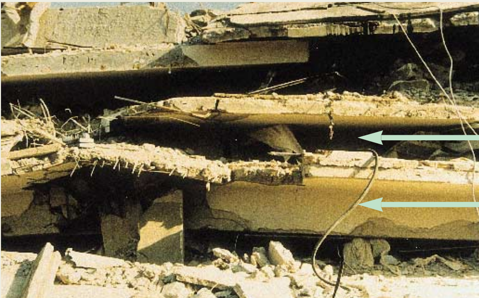
Photo 4: The beams of the ceiling on the front of the ruined building are in contact with the floor slabs. The height of free space right behind the beam is about 40cm. There was information from a tenant that before the earthquake there were people in the living room, to which beam 'A' belongs. There was no sign of survivors.
