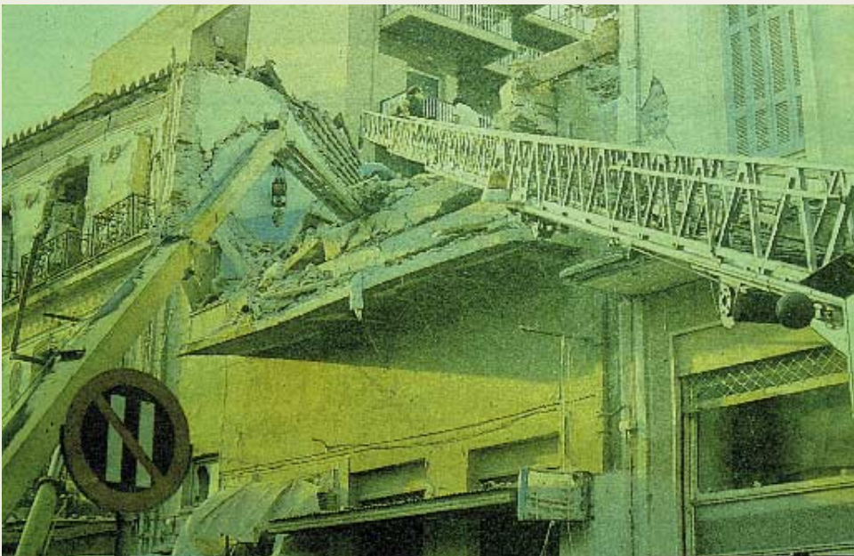
Photo 16: Rescue of trapped persons from a three-storey building of which only the two upper floors collapsed. The risk for the trapped and the rescuers is obvious in case of a possible collapse of the ground floor during a strong aftershock. The crane arm on the left side aims at preventing the collapse of the wall of the near-by building towards the rescue operation front. (Rescue Operation, Kalamata 1986)
