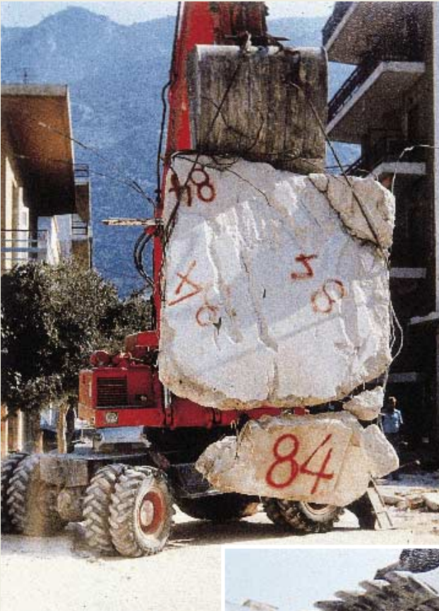
Photo 9-10: Elevation of a slab (photo 9) and a beam element (photo 10) by a shovel excavator. Eccentric fastening so that the main reinforcement takes a vertical direction and therefore the folding of the element is avoided. (Investigation work, Loutraki 1981)
