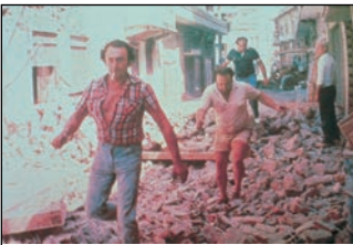
At Kalamata commercial centre, 1986 earthquake
