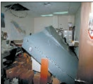
Typical case of unfastened bookshelves falling in offices after an earthquake.
