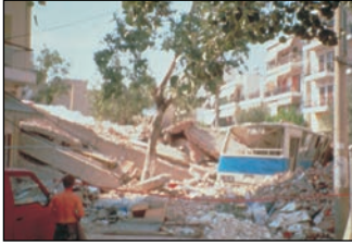
Menidi, (Greece) after the 1999 Parnitha earthquake.
