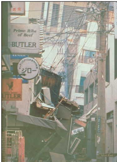
Downtown Kobe, Japan, 1994 earthquake
