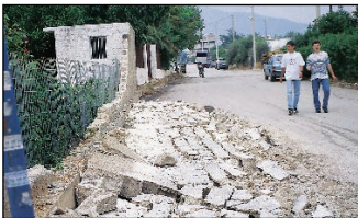
Collapse of a fence in Menidi caused by the 1999 Parnitha earthquake.
