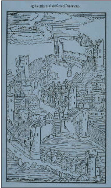
Extended damages in the city of Rhodes (Greece) from the May 3rd, 1481 earthquake (woodcut, 1496, Ulm, Germany). (Source: National Information Service for Earthquake Engineering, University of California, Berkeley, Kozak Collection, http://www.berkeley.edu/cgi-bin/kozak ).
