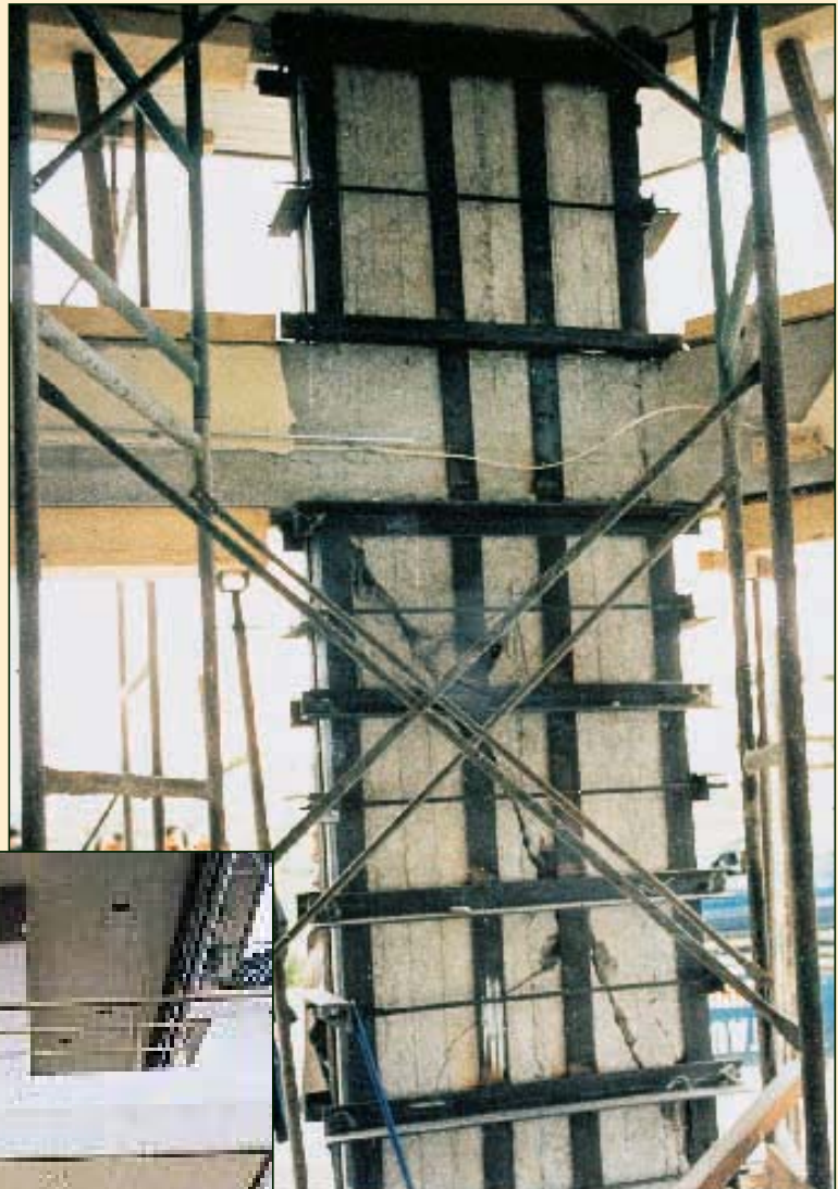
Pyrgos 1993 Propping using tightening procedure
