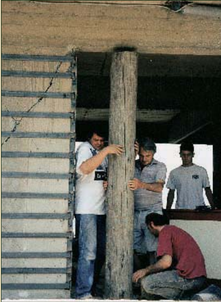
Egion 1995. Tightening using metal plates.
