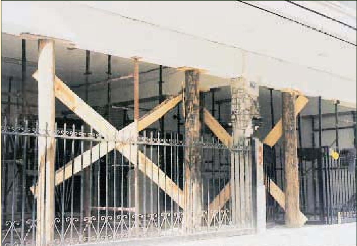
Attika – Ano Liosia 1999 Propping using tree trunks
