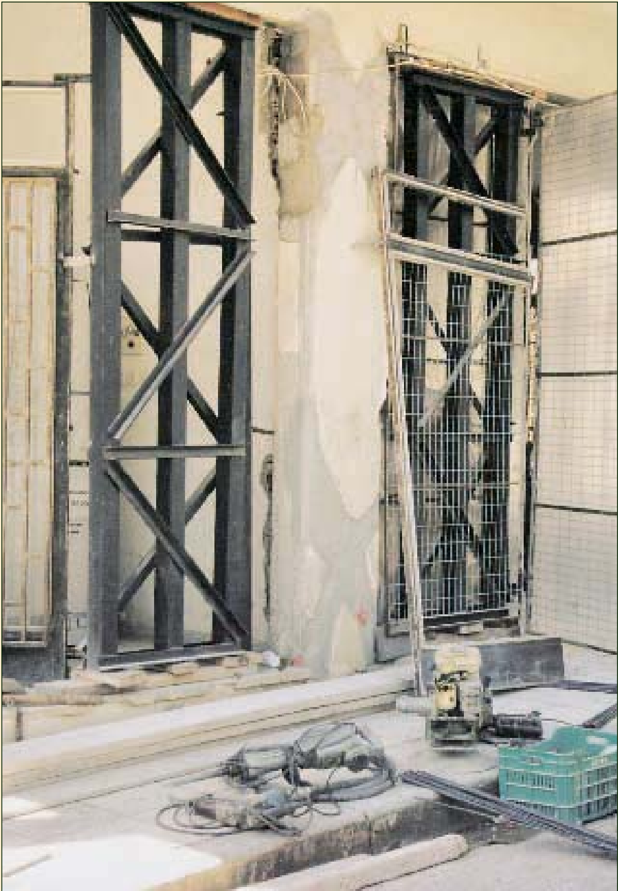
Egion 1995 Propping with square whole section metal beams.
