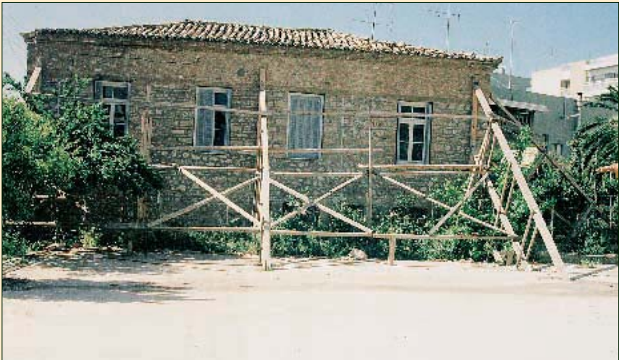
Egion 1995 Shoring using industrial timber
