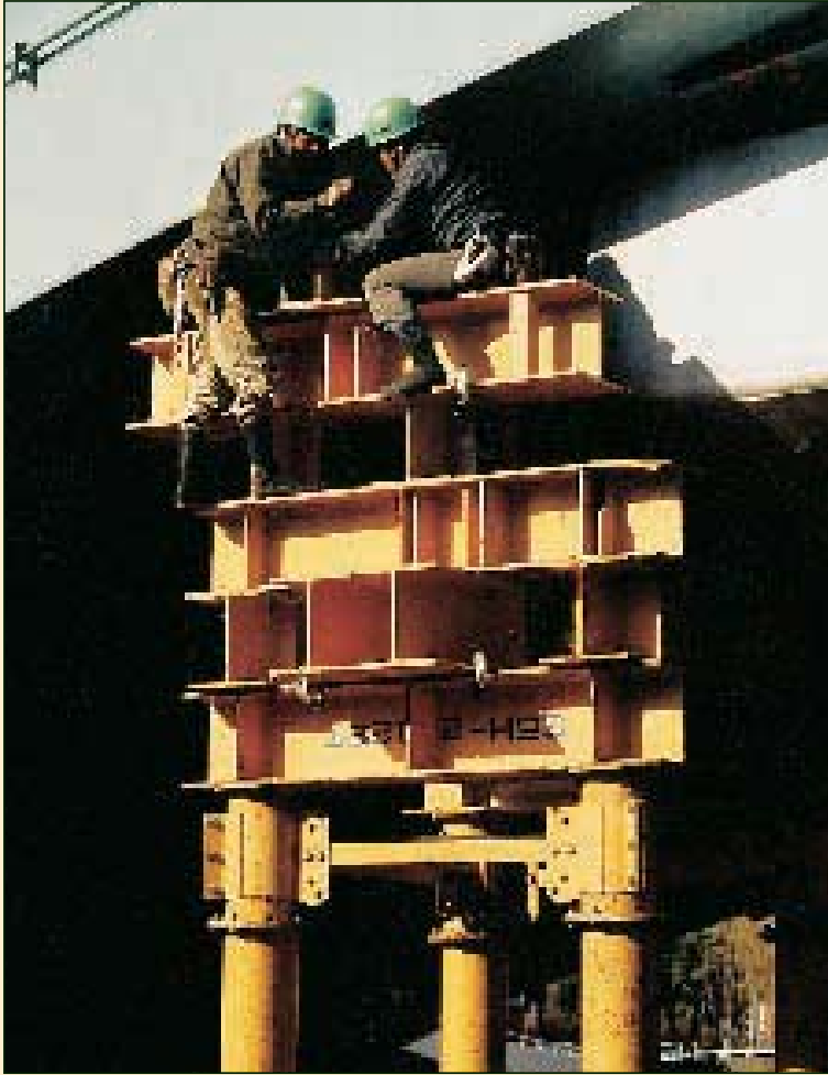
Kobe – Japan 1995 Extended and heavy propping with all sorts of metal sections, heavy type, on big bridges.
