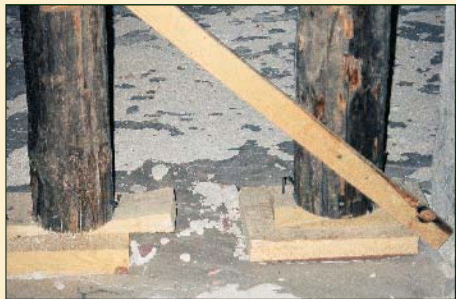
Details of wedging on propping with tree trunks.
