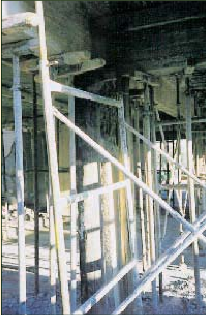
Paphos – Cyprus 1995 Temporary dense propping with metal scaffolding.
