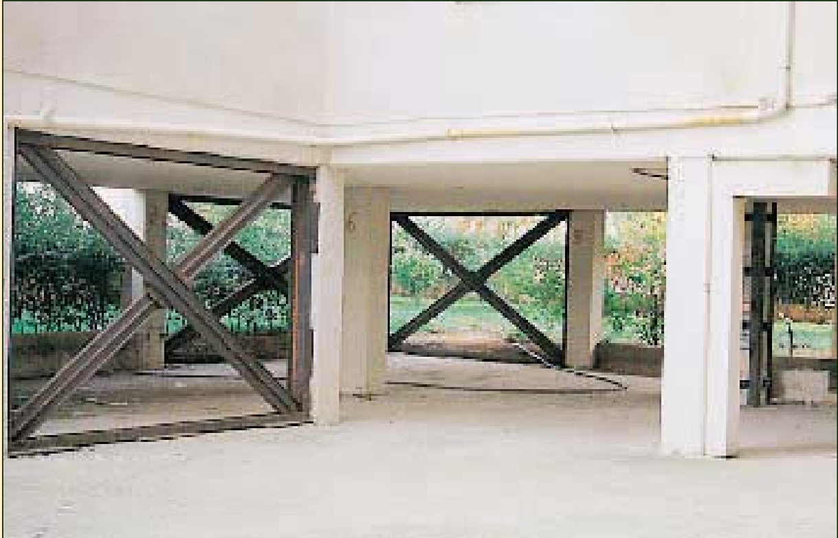
Metamorfosis – Attika 1999 Extended heavy propping with metal plates on damaged pilotis columns.
