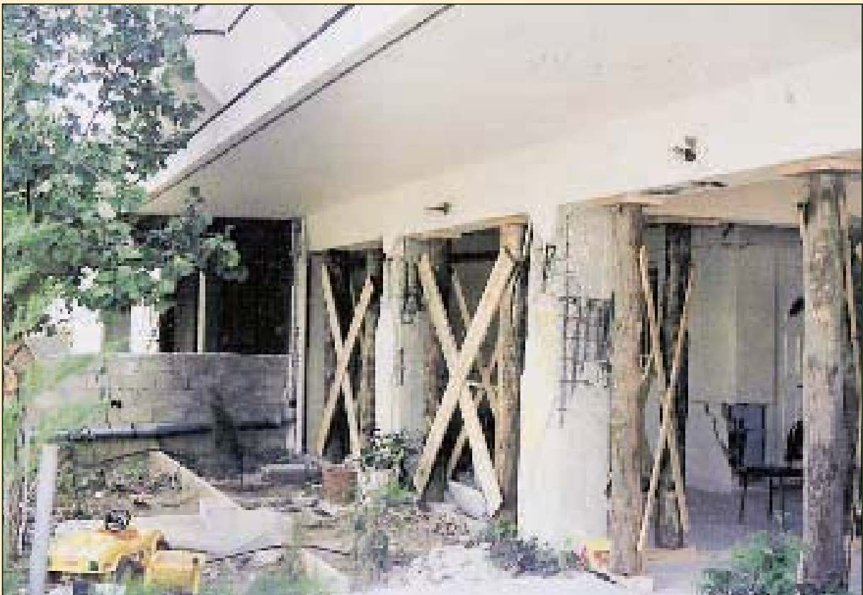
Attika Ano Liosia 1999 Propping with tree trunks.
