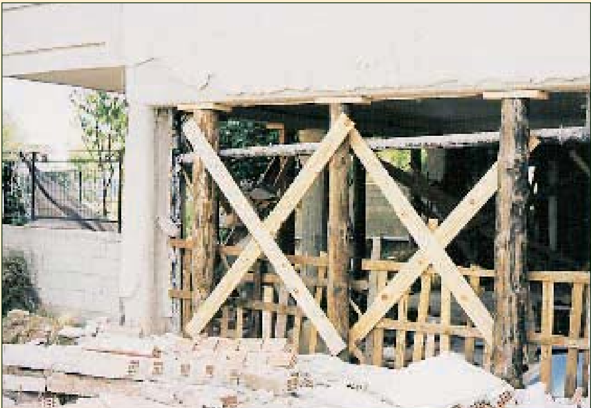
Attika – Ano Liosia 1999 Propping using tree trunks
