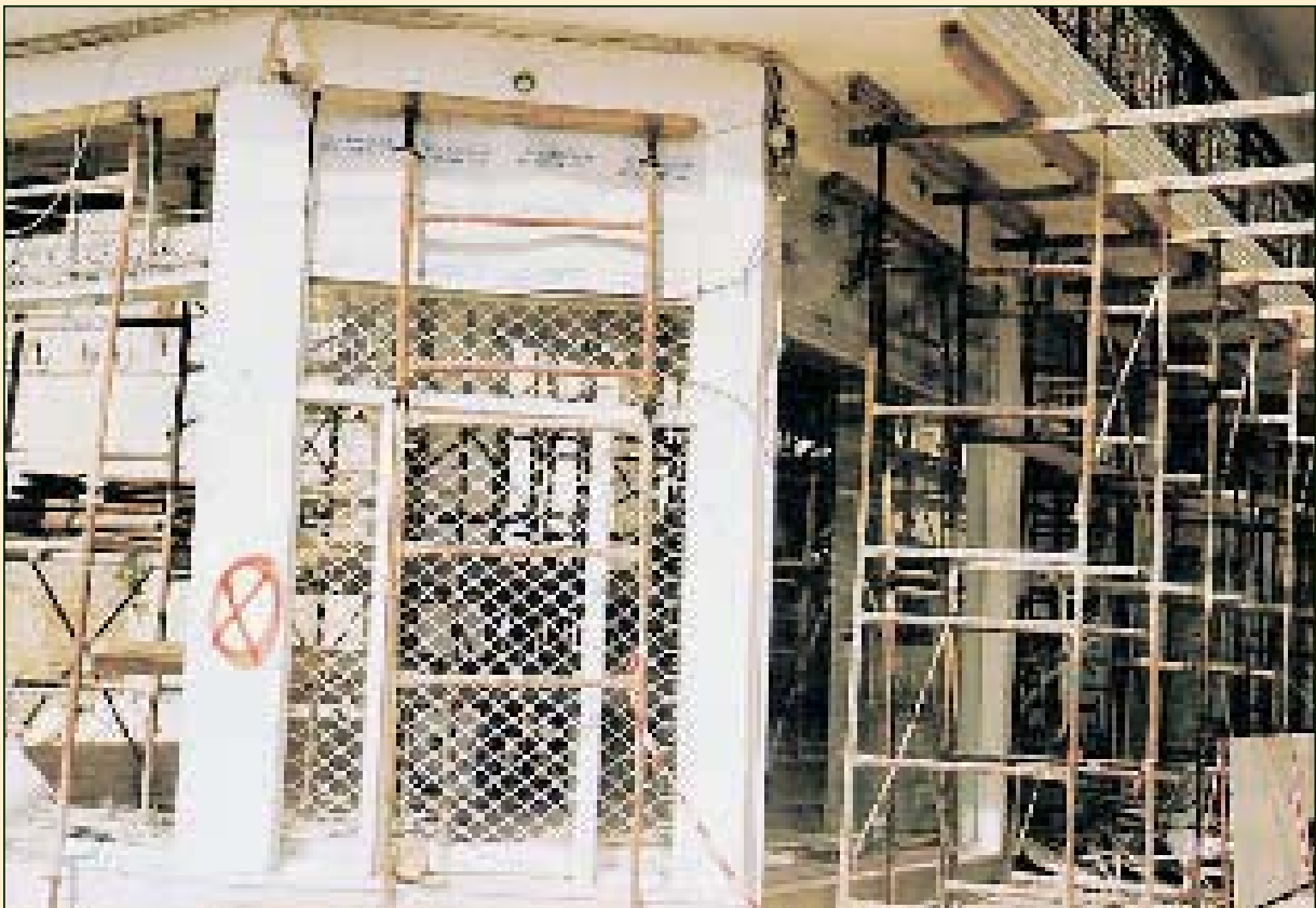
Attika – Ano Liosia 1999 Propping using industrial scaffolding. Their use was extensive in Athens earthquake and in most cases it was proven wrong
