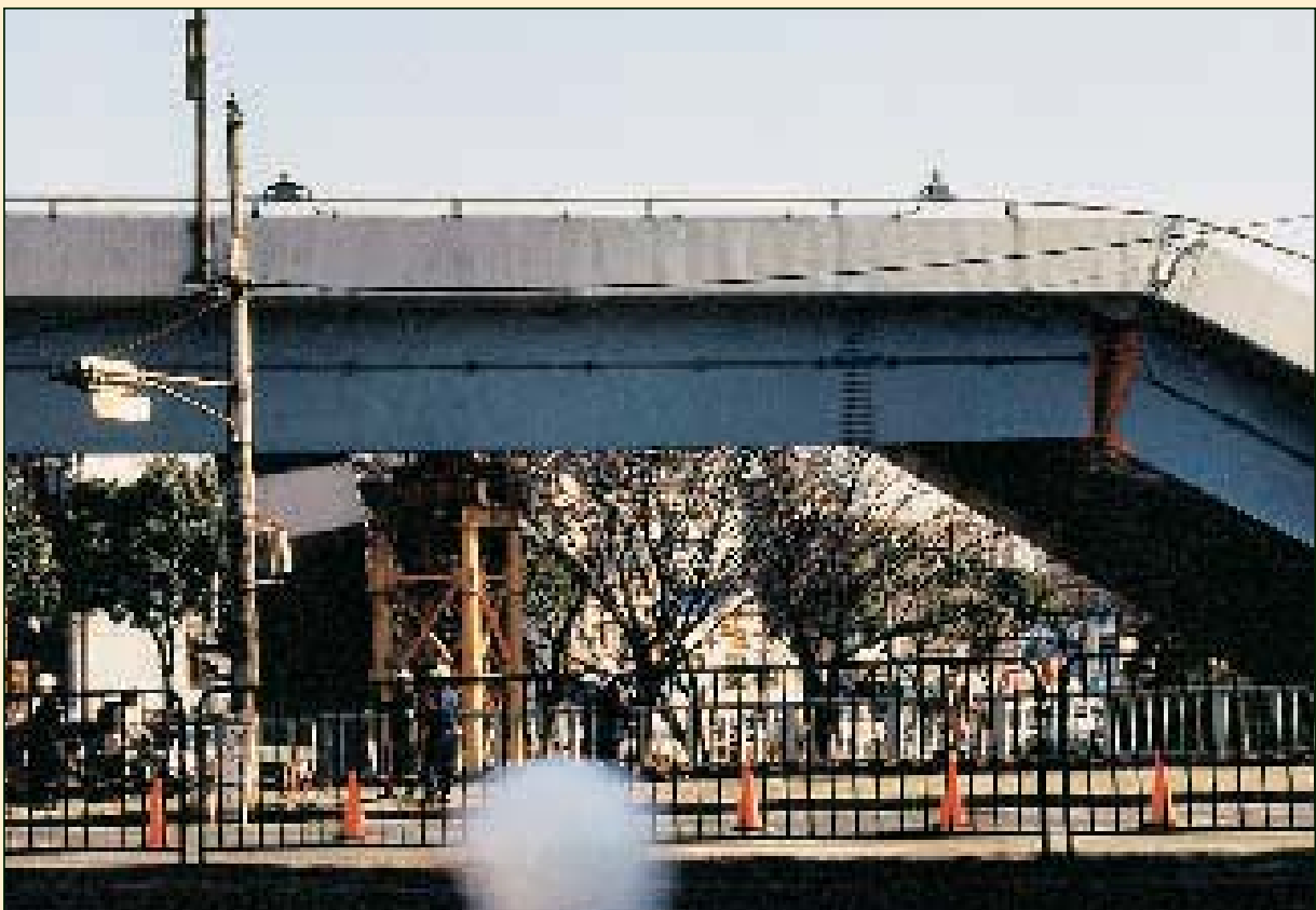
Kobe – Japan 1995 Extended and heavy propping with all sorts of metal sections, heavy type, on big bridges.
