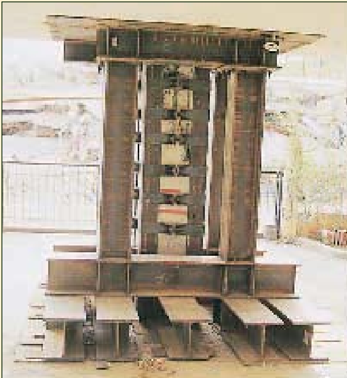
Metamorfosis – Attika 1999 Extended heavy propping with metal plates on damaged pilotis columns.
