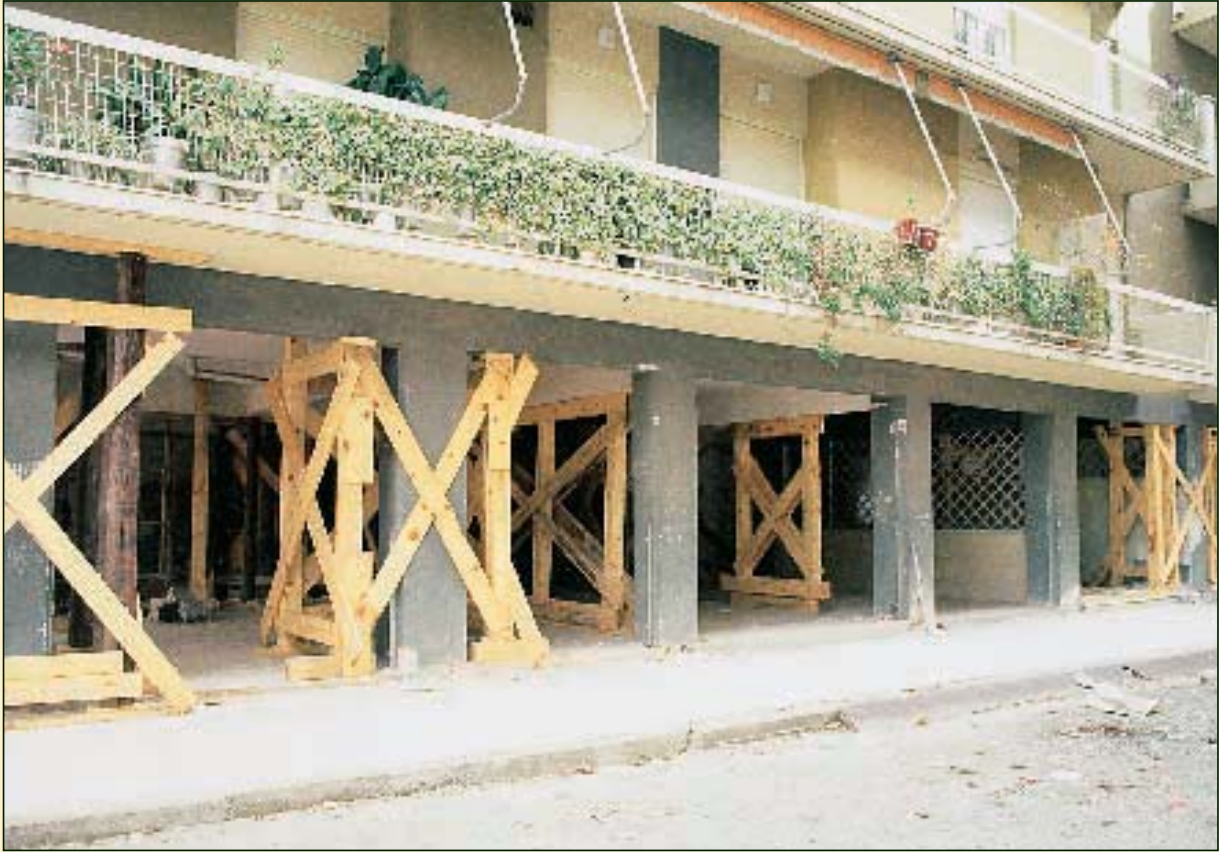
Kalamata 1986 Propping – shoring using industrial timber
