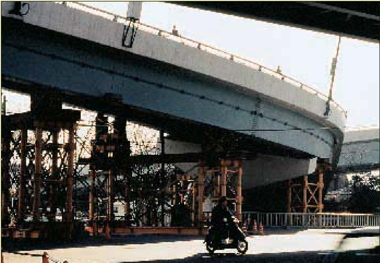
Kobe – Japan 1995 Extended and heavy propping with all sorts of metal sections, heavy type, on big bridges.
