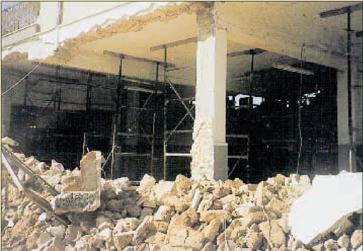
Attika – Ano Liosia 1999 Propping using industrial scaffolding. Their use was extensive in Athens earthquake and in most cases it was proven wrong
