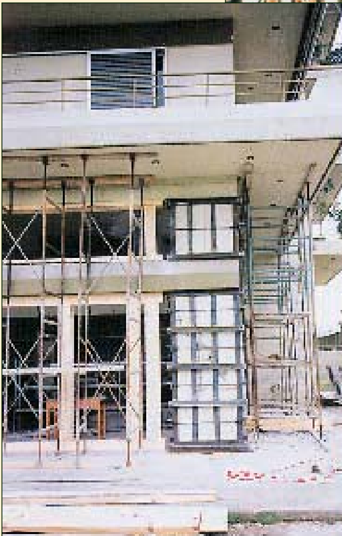
Pyrgos 1993 Propping using tightening procedure
