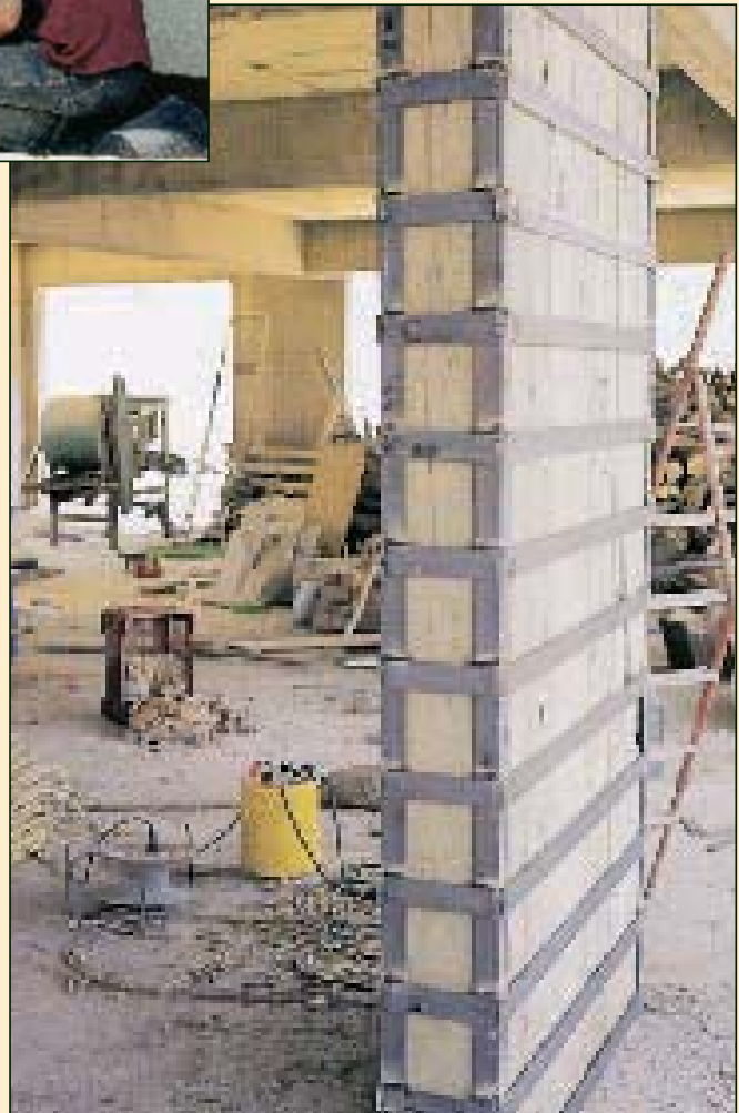
Egion 1995. Tightening using metal plates.
