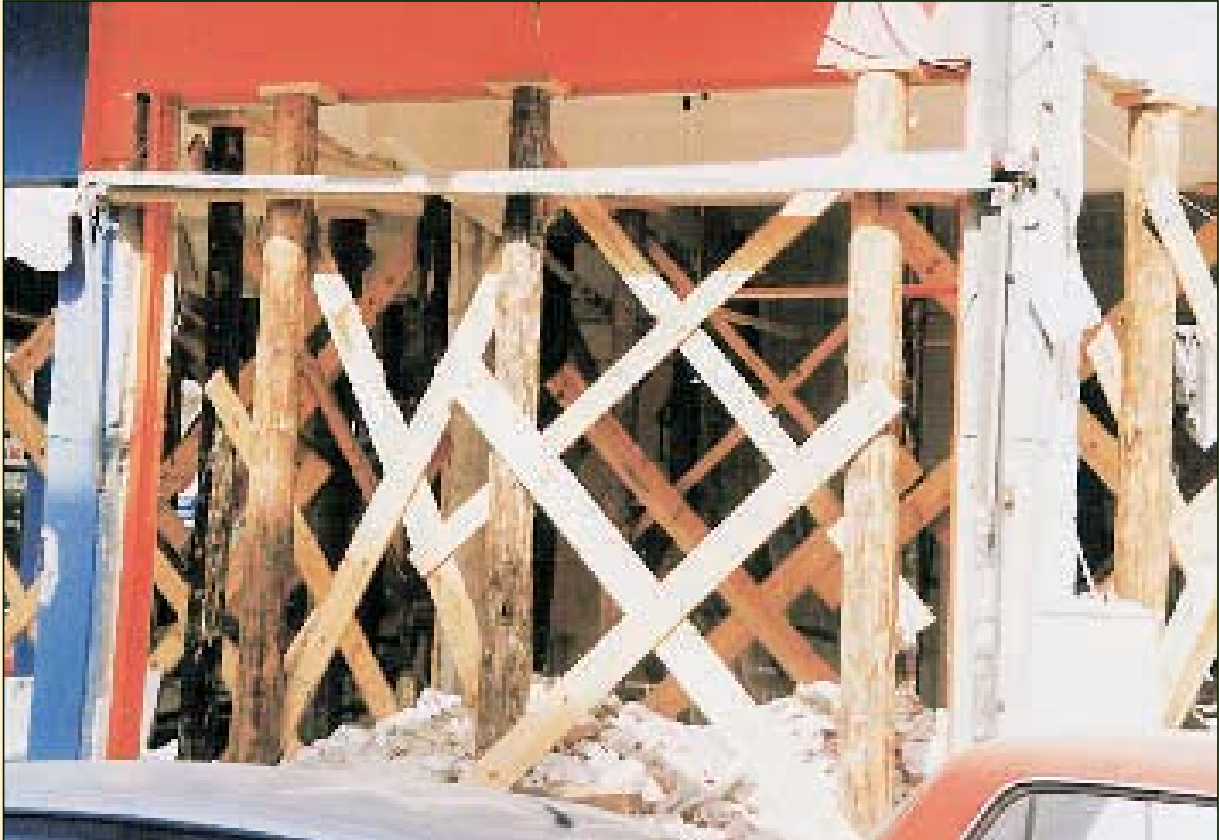
Attika Ano Liosia 1999 Propping with tree trunks.
