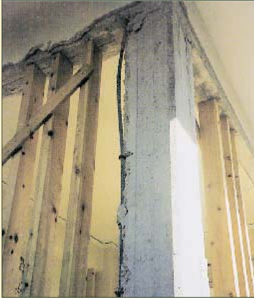
Attika – Ano Liosia 1999. Propping with industrial timber and frames between columns.
