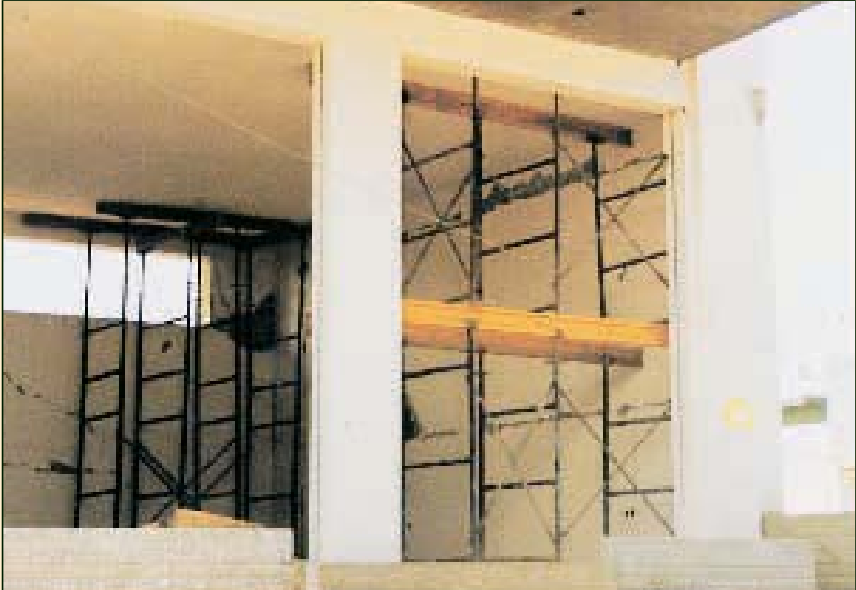
Attika Menidi 1999. Partial propping with scaffolding in pilotis with small damages.
