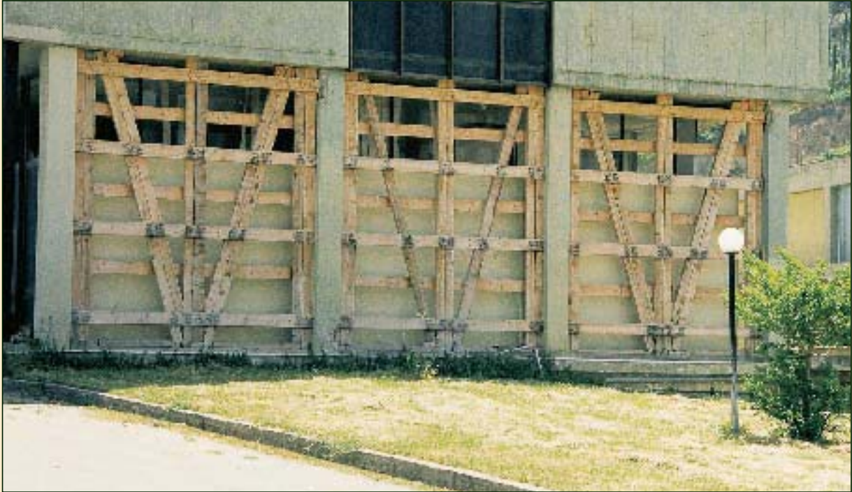
Egion 1995 Perimetric shoring with timber.
